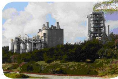
Last year a million tons of cement were produced from the quarried limestone. And Santa Cruz County was dosed in 2006 with 200,000 to 300,000 tons of CO 2 spewed out from that process. Can this local embarrassment be fixed?
